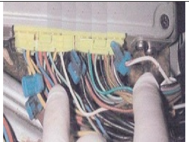
Photo 3-4: Power wire White/Red
