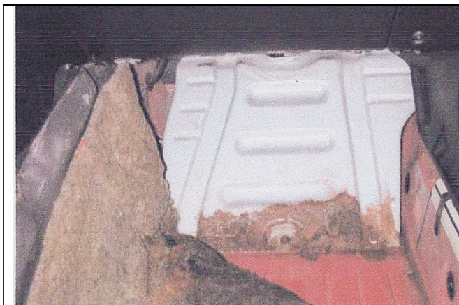
Photo 3-1: ECU Cover on passenger foot well
