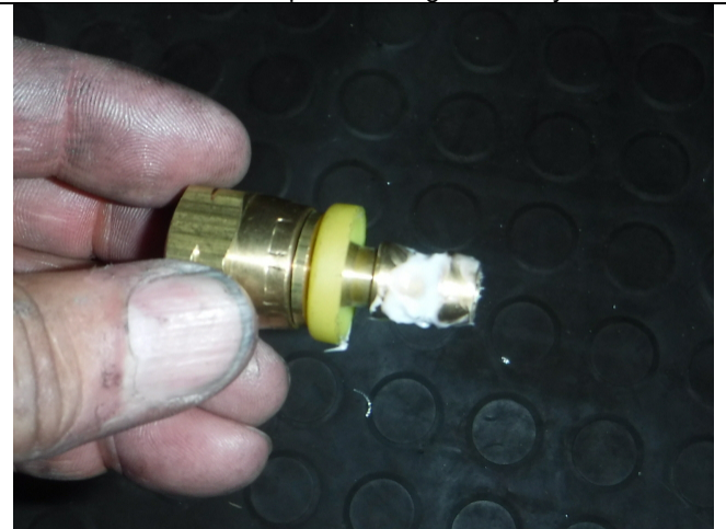
Photo 11-6: Grease applied to the fitting
