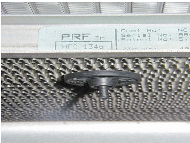
Photo 17-10: Locking clip installed. Note pad should be installed on the condenser coil.
