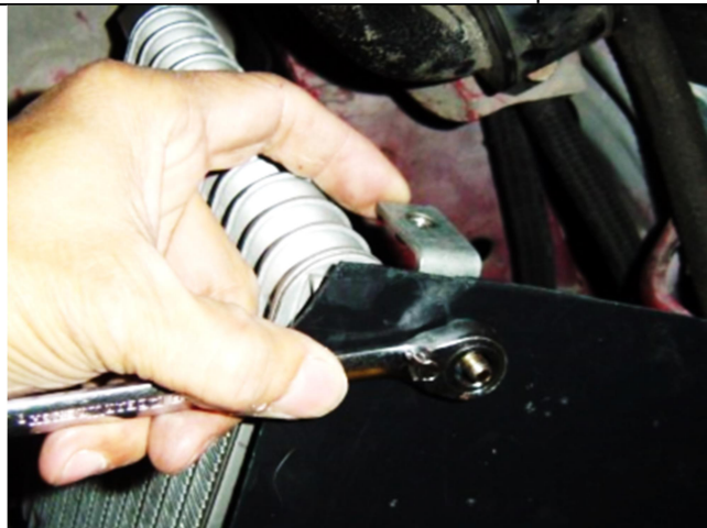
Photo 11-22: Installed L-bracket with nut
