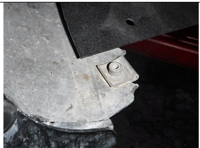
Photo 11-14: Install upper bolts
