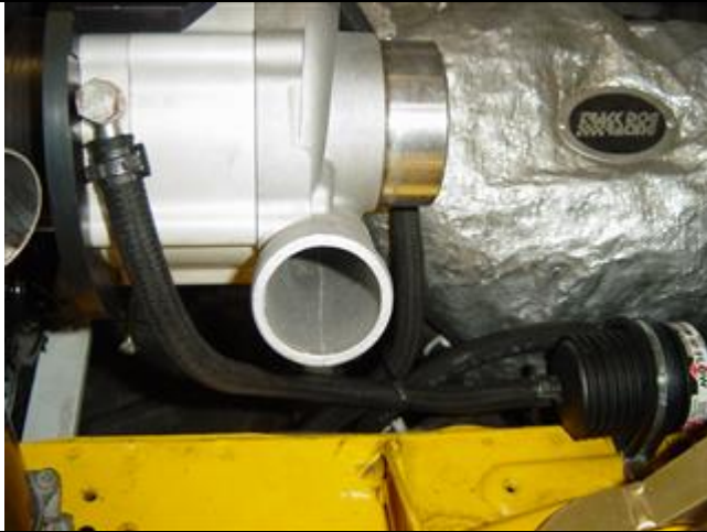
Photo 13-19: Hose installed from filter to SC
