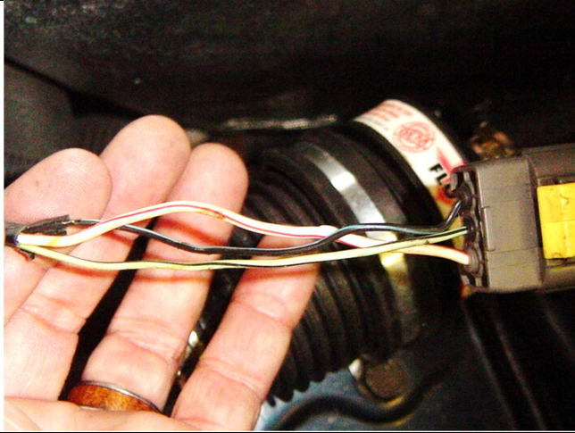
Photo 19-3: Tape removed from harness
