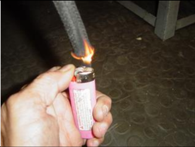
Photo 11-7: Apply heat to soften the rubber
