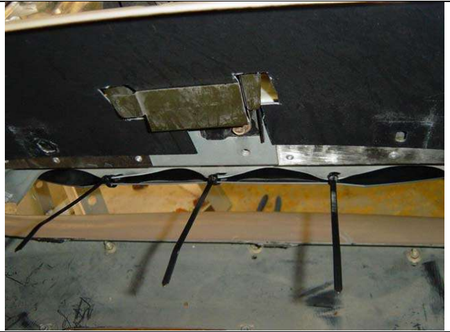
Photo 6-12: Upper 1 panel tie-wrapped to tabs
