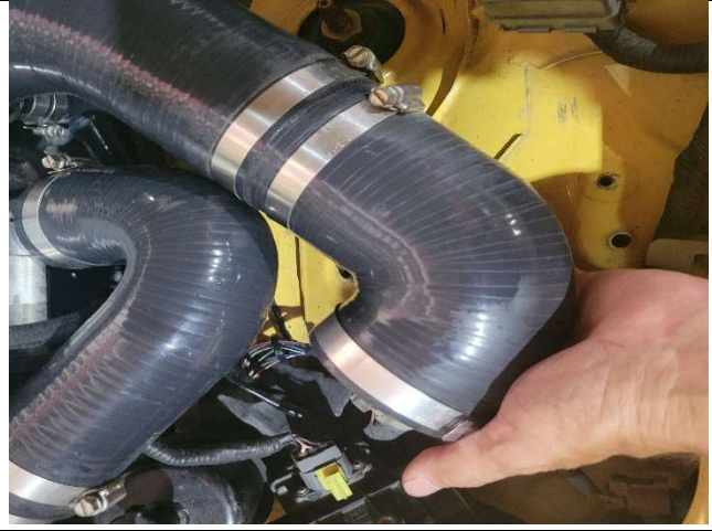
Photo 20-22: 90 degree hose installed
