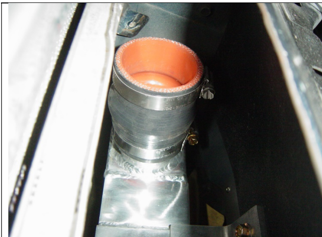
Photo 20-1: Hose installed with clamps
