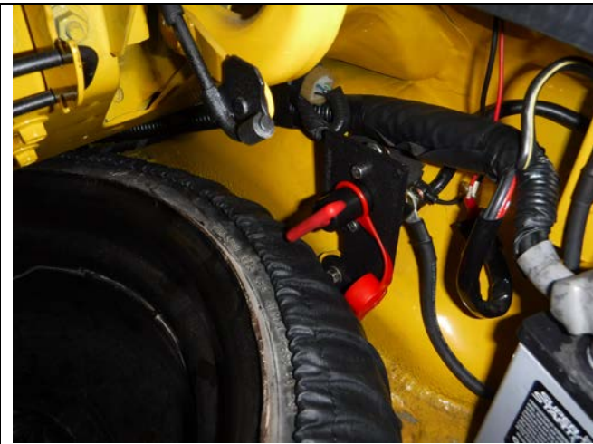
Photo 2-9: Spare tire near the disconnect switch
