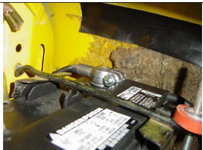
Photo 3-8: Ground strap installed on battery post
