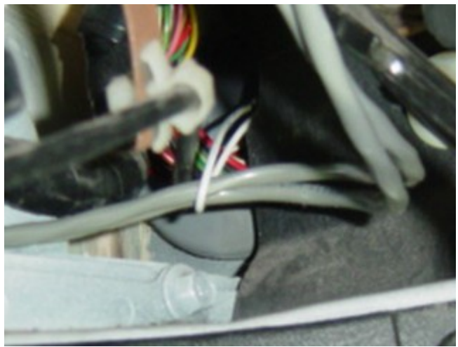
Photo 5-D: Pull the Sensor cables about 12" through the coat hanger loop
