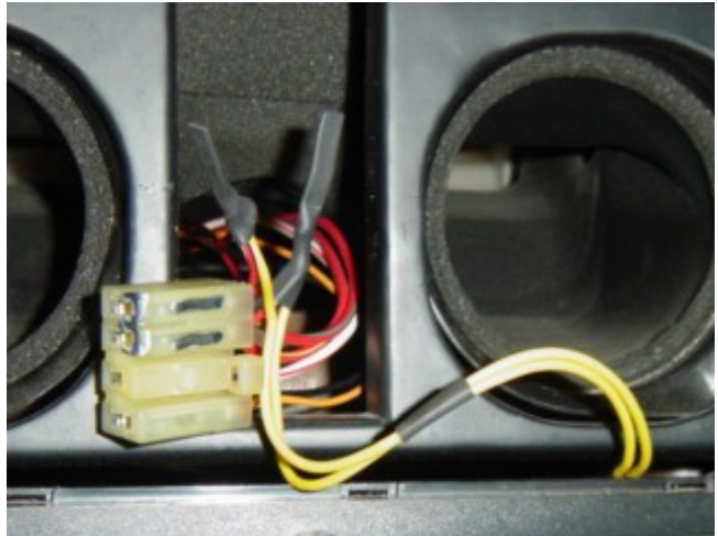
Photo 6-F: Lighting wire soldered to the connector
