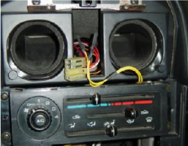
Photo 6-E: Lighting wire pulled behind A/C panel on the right side
