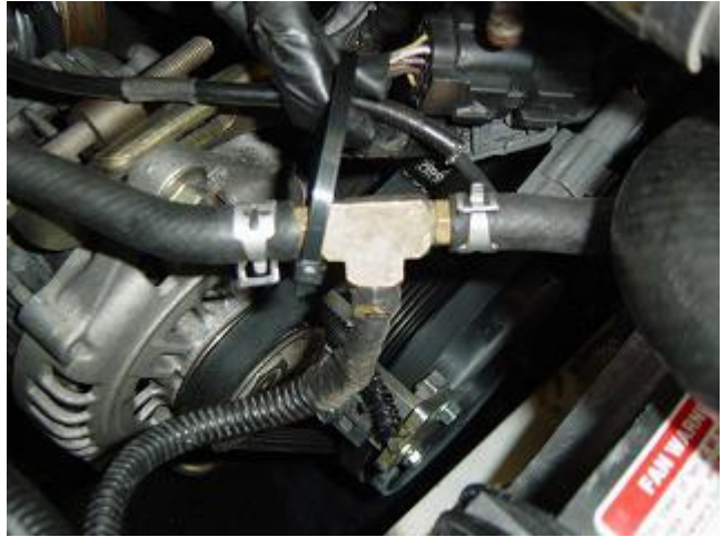
Photo 9-B: Water temperature comes from the Tee provided into the 5/16" hose
