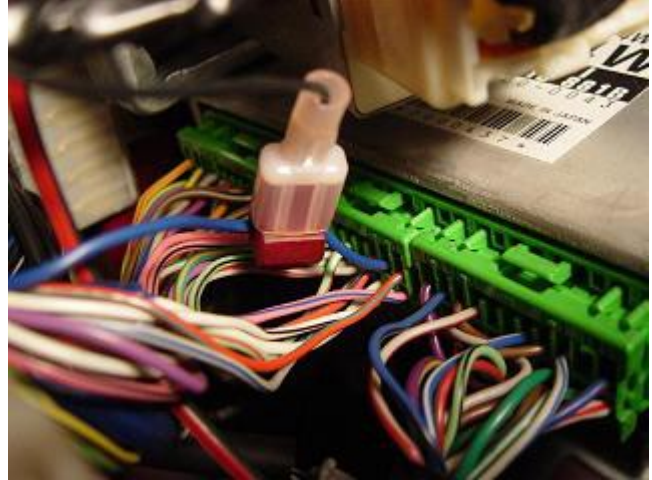
Photo 6-B: Close up of the blue lead wire
