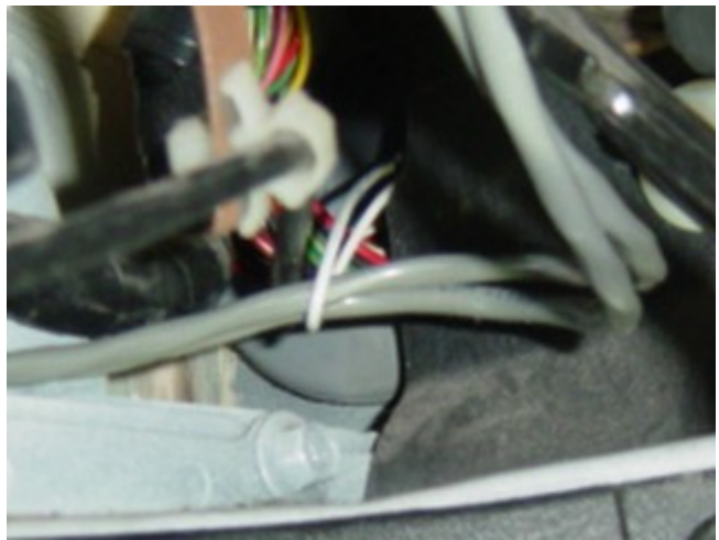
Photo 4-D: Pull the Sensor cables about 12" through the coat hanger loop
